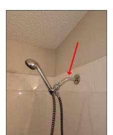
Shower mast is loose in the wall. Recommend securing properly to the wall.
