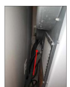
Recommend replacing flexible dry vent pipe and run continuous solid metal pipe. Install solid metal pipe with foil tape, NOT screws or duct tape.
