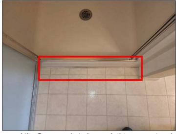
The joint along the shower and the floor needs to be sealed to prevent moisture penetration. Have a contractor evaluate and service as needed.
