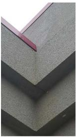
The EIFS wall covering is peeling and cracking, have a contractor evaluate and service as needed.
