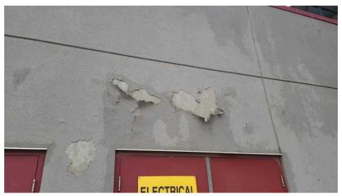
The EIFS wall covering is peeling and cracking, have a contractor evaluate and service as needed.
