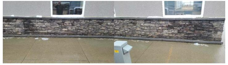
The stone veneer is very loose in places and will need to be serviced. The stone veneer is very loose in places and will need to be serviced.
