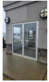
The front aluminum door does not open and will need to be serviced by a contractor.
