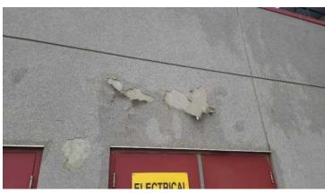
The EIFS wall covering is peeling and cracking, have a contractor evaluate and service as needed.
