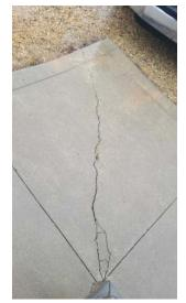
The sidewalks have typical cracks that indicate movement of the base under the sidewalk, water management needs to be addressed to control movement. If this is left it can effect the components of the building and surrounding areas.
