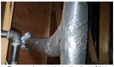
There are pipes penetrating thru the roof that need to be insulated inside to keep the hot and cold air away from each, if not serviced this can cause condensation damage to the the ceiling inside the building. Have a contractor evaluate and service as needed.
