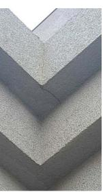
The EIFS wall covering is peeling and cracking, have a contractor evaluate and service as needed.
