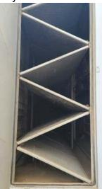
The exhaust system for the warehouse area has a The exhaust systems are very dirty and should be few leaking that should be serviced by a serviced by a contractor accordingly.
