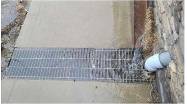
The drainage swales are clogged and leaking back towards the building, there are high levels of moisture in the concrete floor inside the building.
