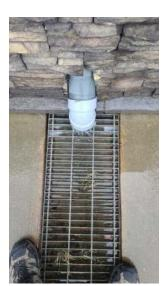
The drainage swales are clogged and leaking back towards the building, there are high levels of moisture in the concrete floor inside the building.
