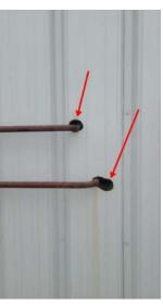
There are holes around some of the pipes in the warehouse area that need to be sealed.
