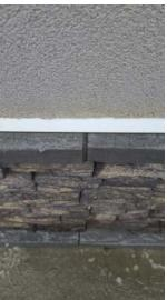
The stone veneer is very loose in places and will need to be serviced. The stone veneer is very loose in places and will need to be serviced.
