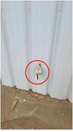
There are loose outlets on the outside of the building, have an electrician service these accordingly
