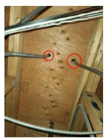
There are pipes penetrating thru the roof that need to be insulated inside to keep the hot and cold air away from each, if not serviced this can cause condensation damage to the the ceiling inside the building. Have a contractor evaluate and service as needed.
