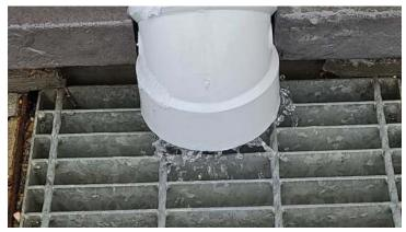
The drainage swales are clogged and leaking back towards the building, there are high levels of back towards the building, there are high levels of moisture in the concrete floor inside the building. Have a contractor evaluate and service as needed.
