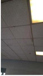
There are signs of moisture in the building that should be monitored, with the grading and drainage being poor this is a problem that may continue. A contractor should be used to evaluate continue. A contractor should be used to evaluate the property and how to keep the moisture away from the building.
