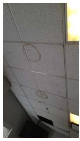
There are signs of moisture in the building that should be monitored, with the grading and drainage being poor this is a problem that may continue. A contractor should be used to evaluateò the property and how to keep the moisture away from the building.
