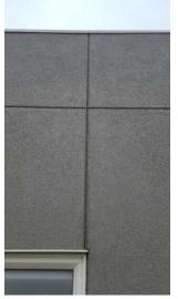
The EIFS wall covering is peeling and cracking, have a contractor evaluate and service as needed.
