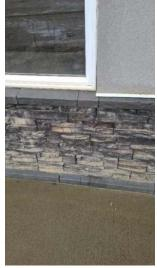
The stone veneer is very loose in places and will need to be serviced. The stone veneer is very loose in places and will need to be serviced.
