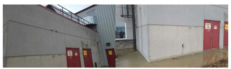
The EIFS wall covering is peeling and cracking, have a contractor evaluate and service as needed.
