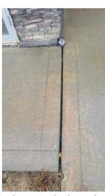
The sidewalks have typical cracks that indicate movement of the base under the sidewalk, water management needs to be addressed to control movement. If this is left it can effect the components of the building and surrounding areas.
